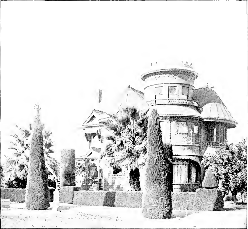
Residence of O. T. Dyer, Manager of the Riverside Banking Company.
